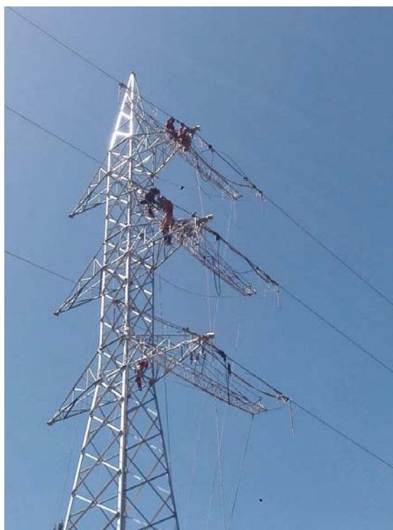
LAT 220kV simple circuito
